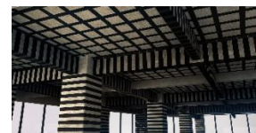
Curing and protecting
