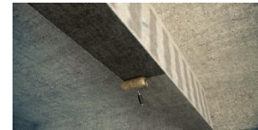
Applying epoxy resin adhesive
