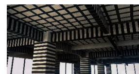
Curing and protecting
