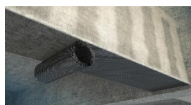
Pasting carbon fiber cloth
