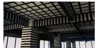
Curing and protecting
