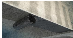
Pasting carbon fiber cloth
