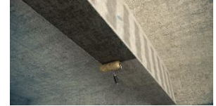
Applying epoxy resin adhesive
