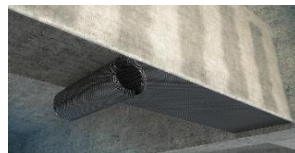
Pasting carbon fiber cloth
